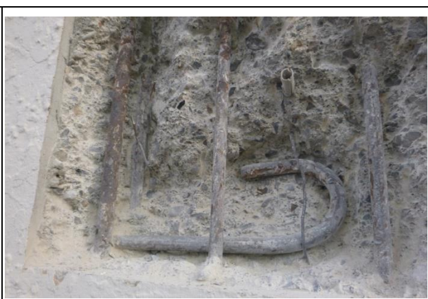
Figure 2: Hook in reinforcing bar found
