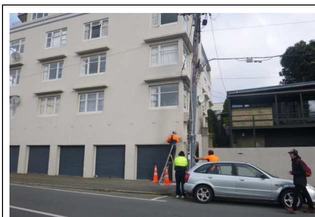
Figure 1: Area of investigation
